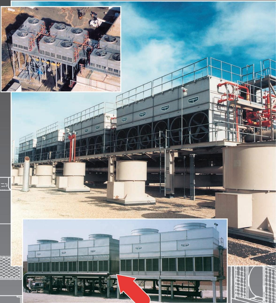
• Reduced Clearance Dimensions with EVAPCO Induced Draft Counterflow Products •
